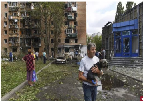
Residents leave an apartment building damaged in shelling by Ukrainian forces in Kursk, Russia, on Aug. 11, 2024. (AP Photo, File) more >
